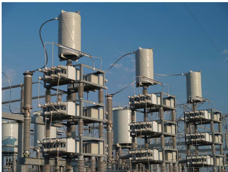
Figure 31. Bank of shunt capacitors used to compensate the voltage at the receiver end of a high-voltage ac transmission line.
