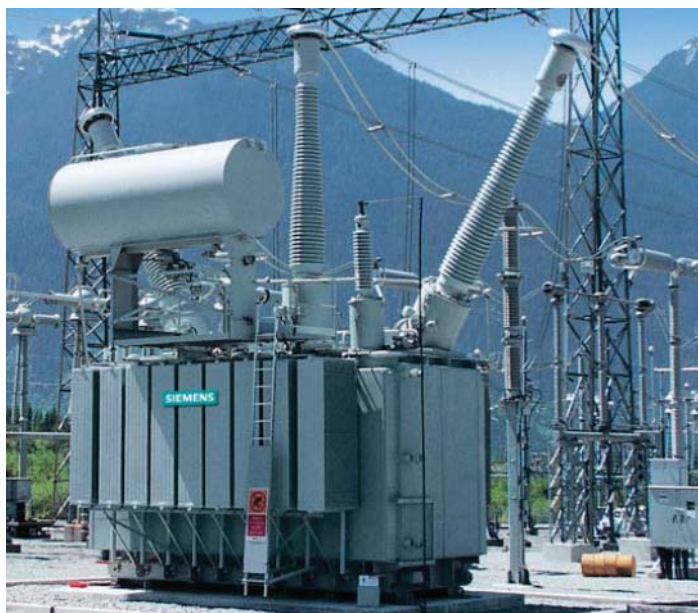
Figure 30. Shunt inductor (three-phase unit) used for voltage compensation of a high-voltage ac transmission line. Each long arm on the top of the unit shown in the picture is an insulator providing access to one end of an inductor (©Siemens AG 2014, all rights reserved).
