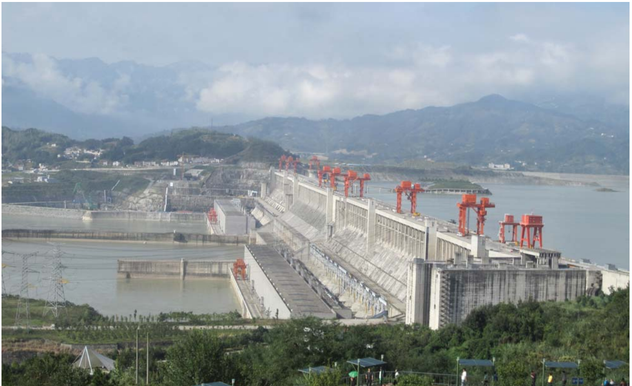
Figure 1-6. Most of the electricity worldwide is produced by three-phase synchronous generators. The above picture shows the Three-Gorges Dam hydropower plant, on the Yangtze River, in China. It contains thirty 700 MW three-phase synchronous generators, each weighing about 6 000 000 kg (about 6000 tons).
